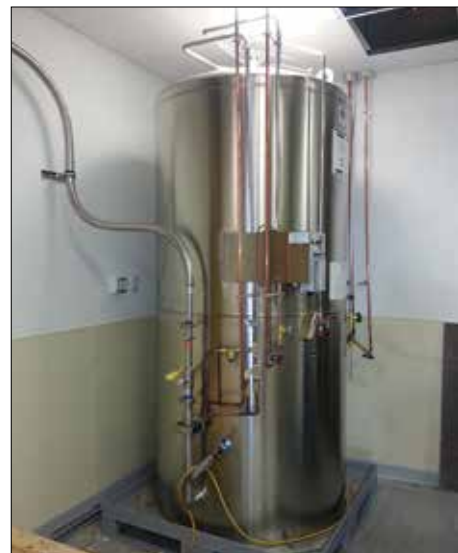
Switching from liquid cylinders (left) to microbulk tanks (right) can save customers space and eliminate the handling of cylinders.
