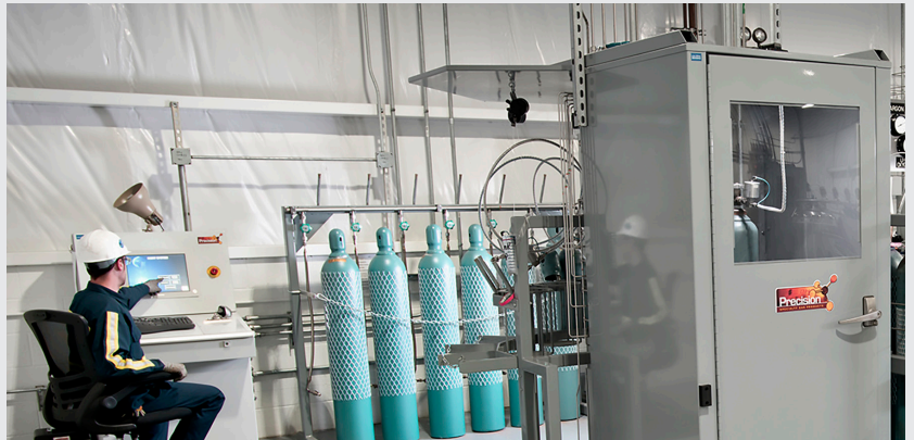
© Weldcoa | Middlesex invested over $1 million in its new automated specialty gas plant
